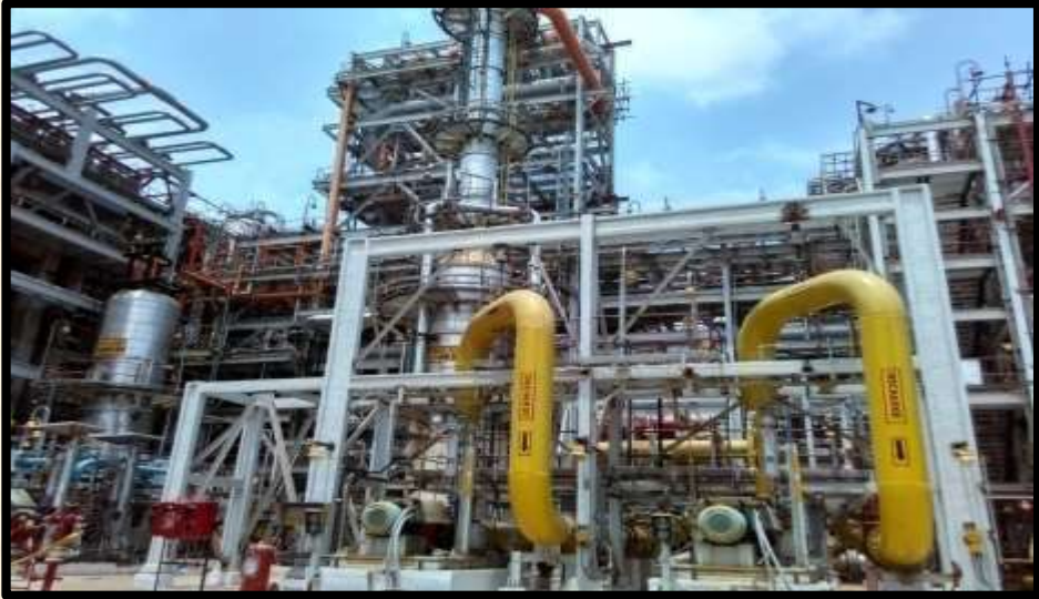
Unit Piping Work at IOCL Paradip Refinery Project
