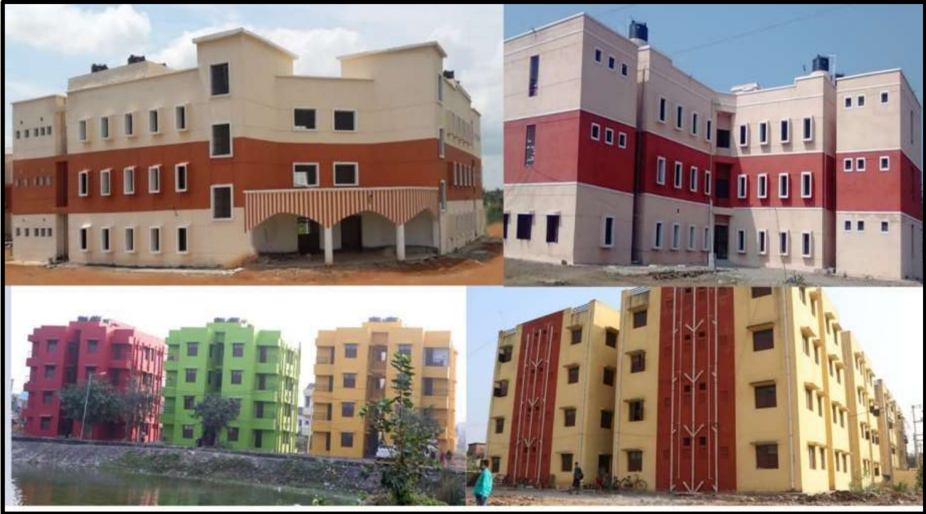
Capital Works for Government of Odisha at various locations Top: Hostels for Tribal Students Under Anwasha Scheme Bottom: Low Cost Housing for EWS
