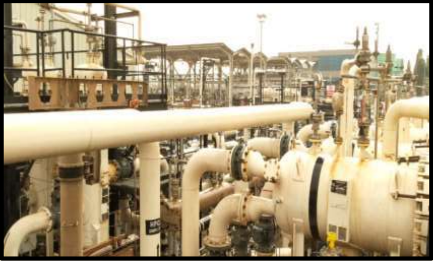
Composite Works for Mumbai Aviation Fuel Farm Facility
