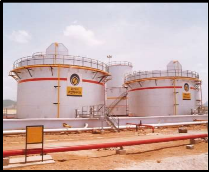
Floating Roof Tanks at BPCL Vijaywada
