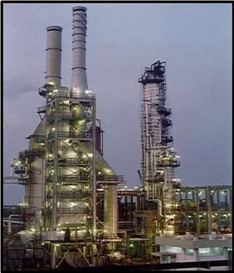
VDU Furnace at IOCL, Haldia
