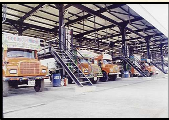
Truck Loading Gantry at IOTL Uran
