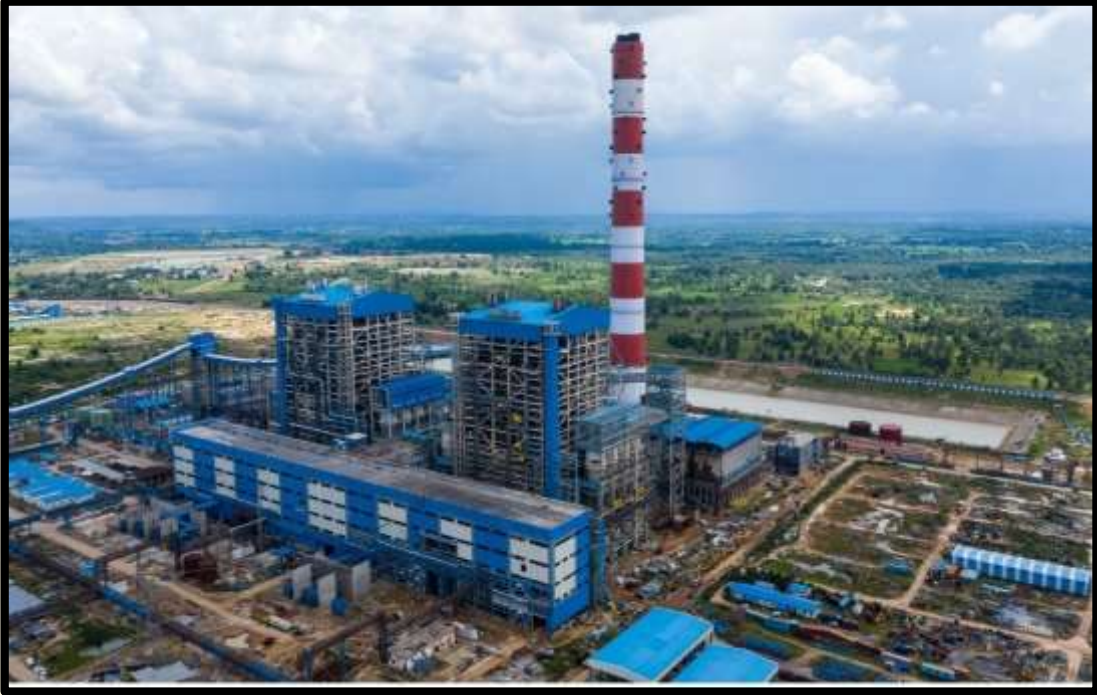
Main Boiler and its Auxiliaries, Piping, Equipment, Bunker & Allied work at NTPC Darlipali 2x800 MW STPP for BHEL
