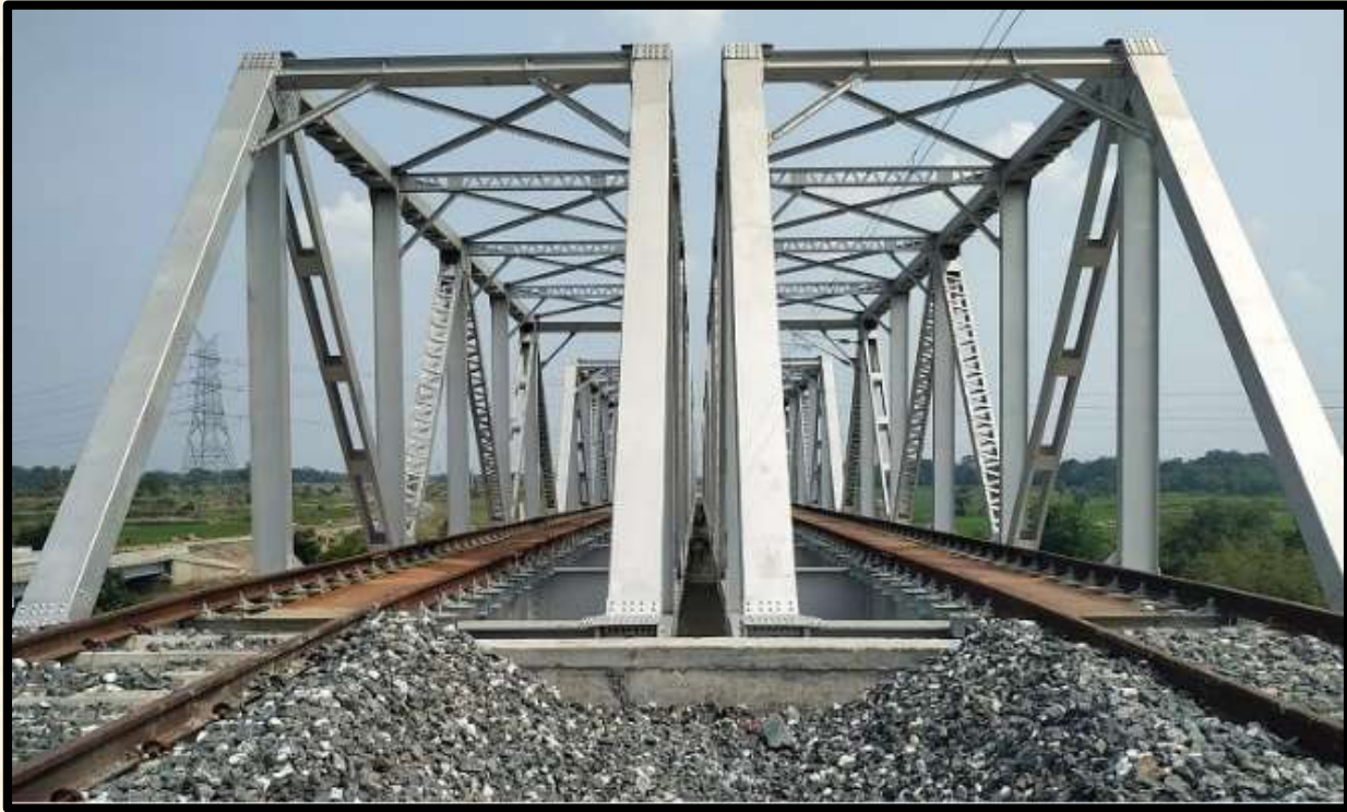
3X2, 30.5 m open web through girder rail bridge over Uthala River at railway siding project of DVC for RITES Ltd. at Raghunathpur
