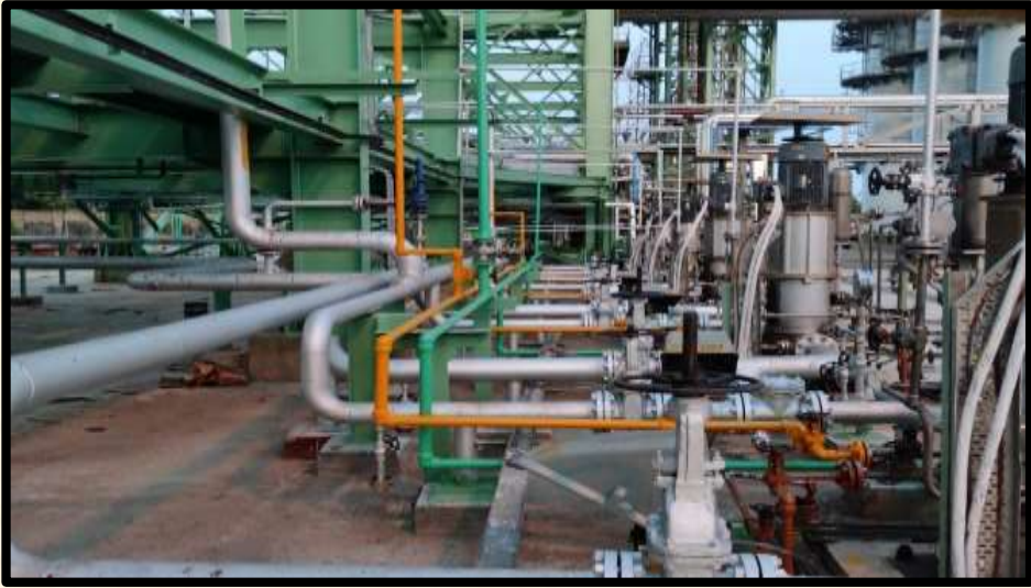
Unit Piping work at CPCL Chennai
