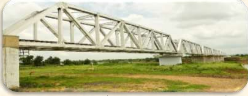
Fabrication and Launching of open web through girders for major bridges between Jhalawar-Aklera section for W.C. Railway
