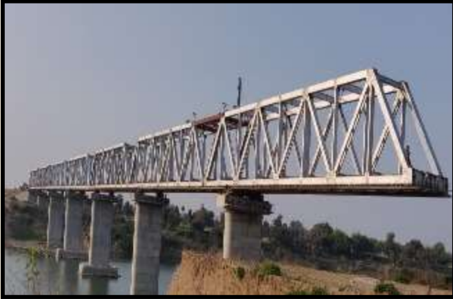
Railway Bridge at Kota for West Central Railway
