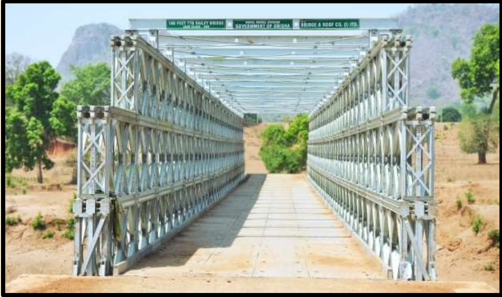
95 Nos. Bailey Type Unit Bridges including approach roads at different locations in Rayagada, Odisha for government of Odisha.
