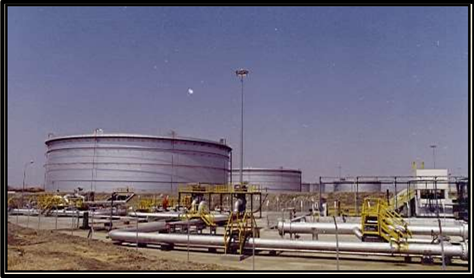
Turnkey Execution of 42,850 KL Oil Terminal for HSD, MS & SKO for IBP at Panipat
