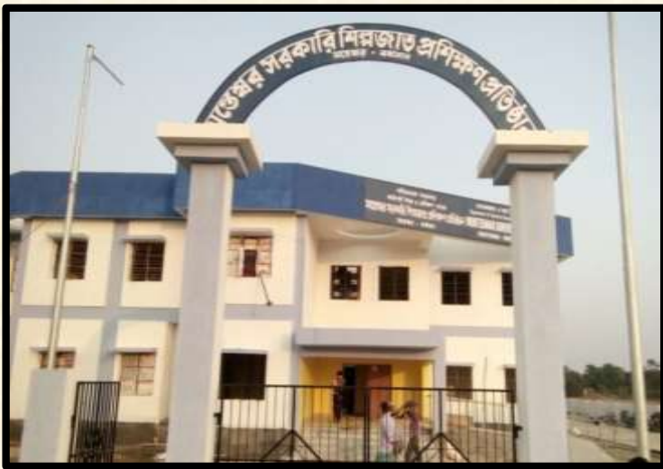
Construction of Industrial Training Institutes / Polytechnics for Govt. of West Bengal, Technical Education and Training Department
