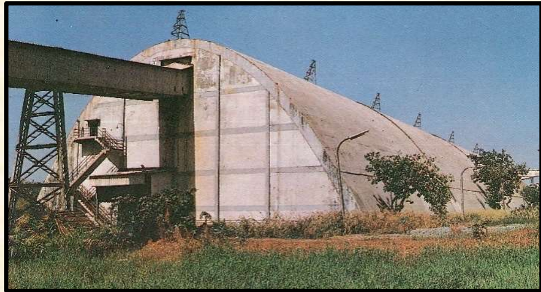
Parabolic RCC Storage Silo for Rashtriya Chemicals & Fertilizers Ltd. at Trombay
