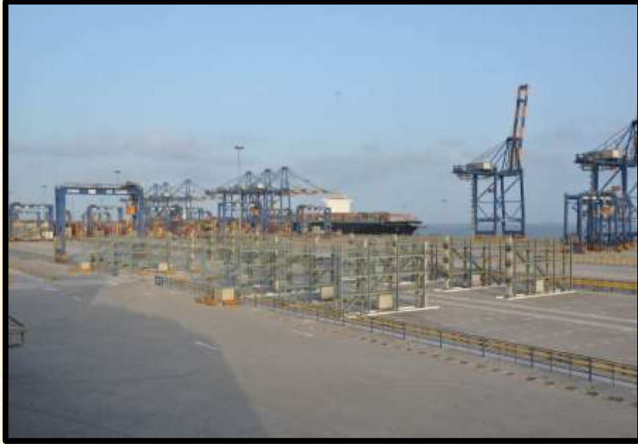
Backup Yard at Adani Mundra Port, Gujarat
