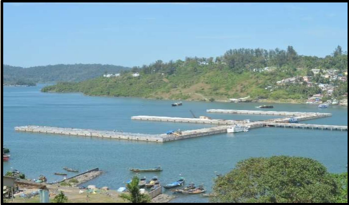
RCC Finger Jetty with Approach at Junglighat Harbour in Port Blair for Andaman Harbour Works
