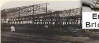
Iron Work (Fabrication & Erection) for East Indian Railways, Lucknow.
