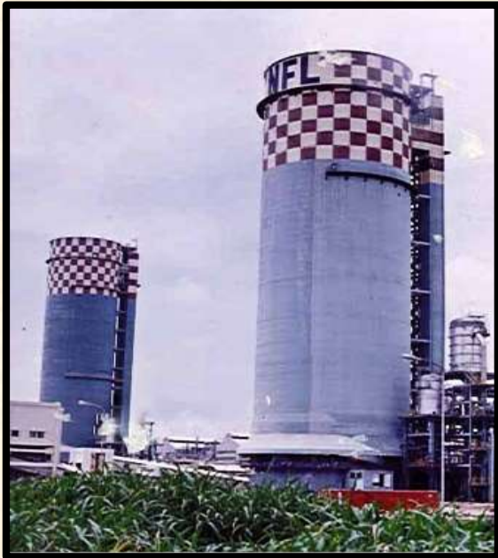
Urea Prilling Tower at National Fertilizers Ltd. Guna
