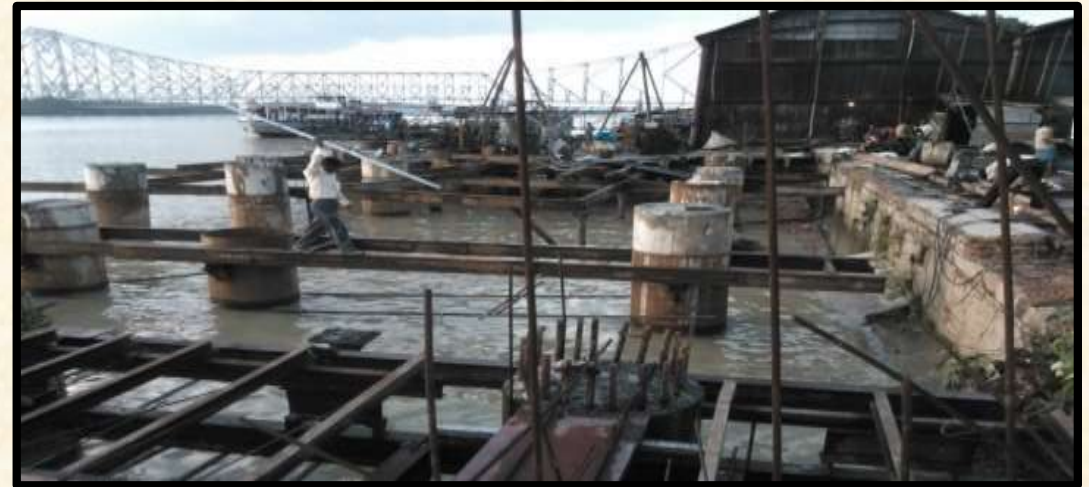
Hooghly River Front Development Work of Kolkata Municipal Corpn.
