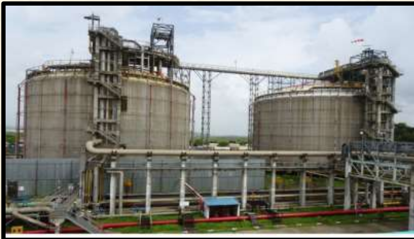
79m dia. Steel Storage Tanks at Hindustan Corpn. Ltd Kanpur Terminal
