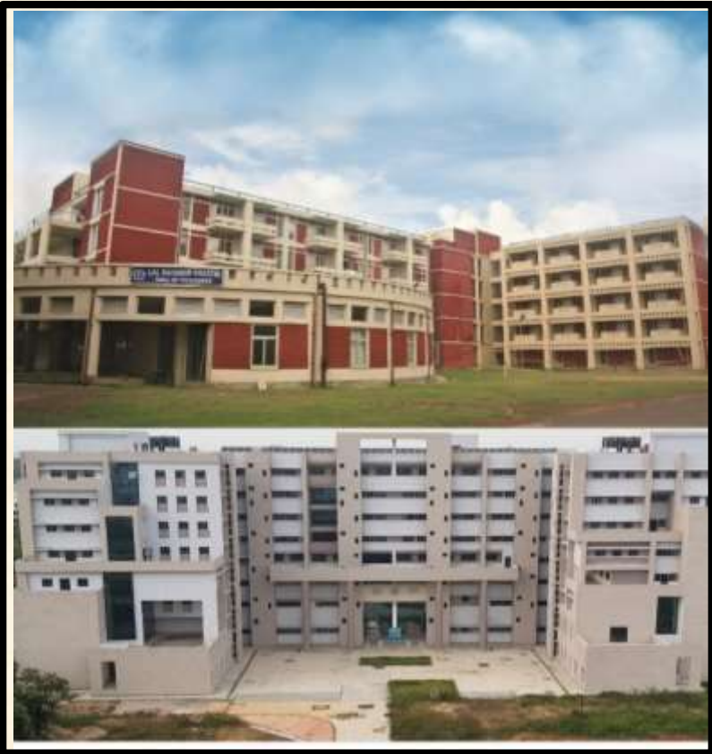
Buildings, Hostels, Residential quarters and other Infrastructure at Indian Institute of Technology, Kharagpur
