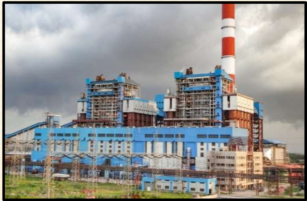
Power Block Unit for 2X500 MW Unit # 1 & 2 at Durgapur Steel Thermal Power Station of DVC at Andal
