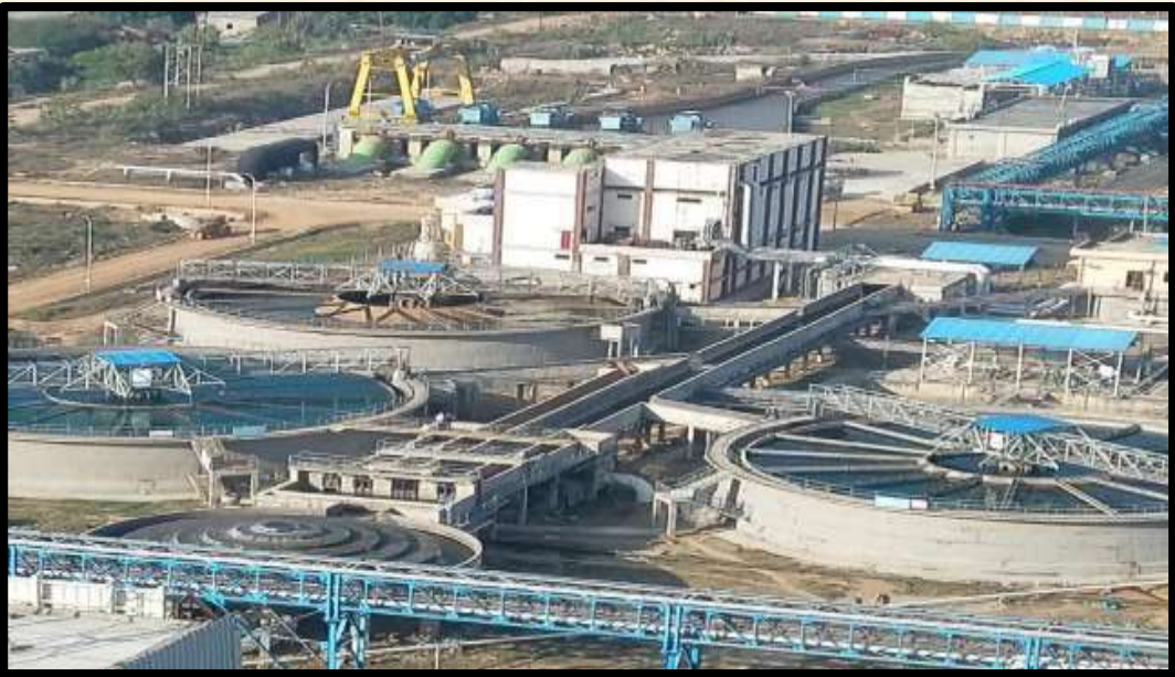
Water Pre Treatment and Liquid Effluent Treatment Plant at MUNPL Meja, Allahabad
