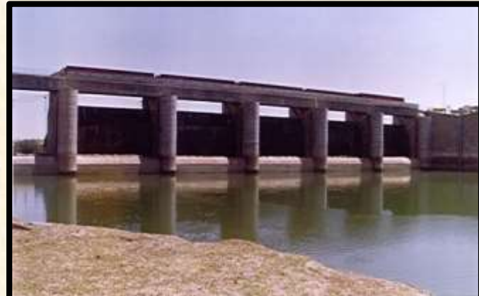
Construction work at Gosunda Dam, Rajasthan of HZL for Tungabhadra Steel Products Ltd.
