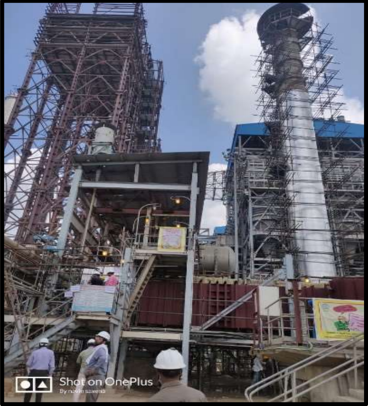
Boiler along with Mill Bunker Structures of North Karanpura 3x660 MW STPP of NTPC for BHEL
