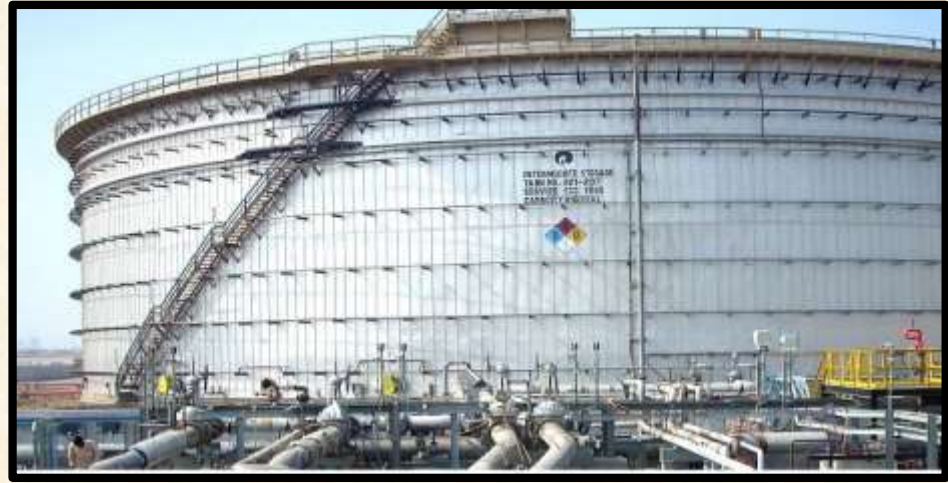
Tanks in RTF unit at Jamnagar Export Refinery Project Reliance Industries Ltd.
