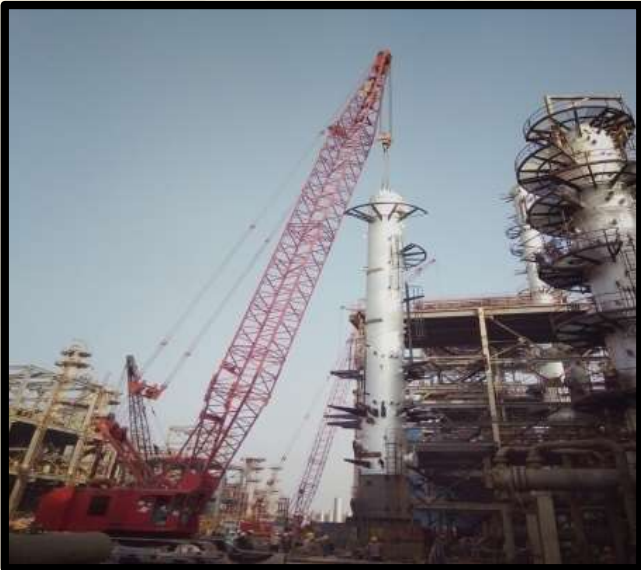
Heavy equipment erection at for Aishwarya Project at IOCL Haldia Refinery
