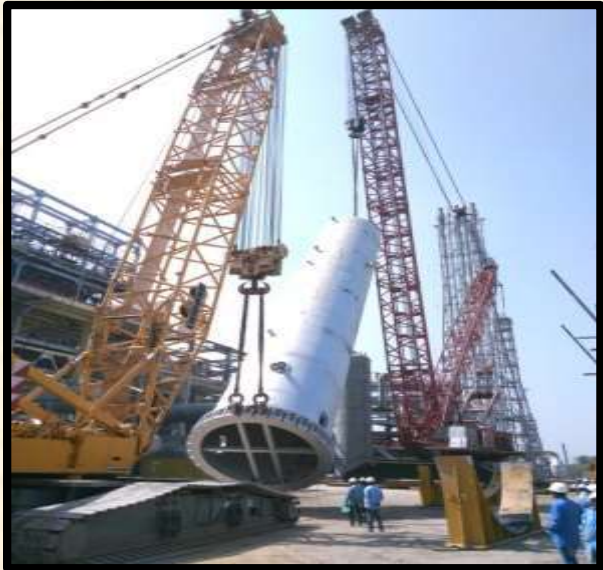
Heavy equipment erection at BPCL Mahul
