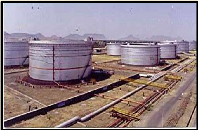
Double Deck floating roof crude oil storage tanks at Indian Oil Corporation Ltd., Mundra.
