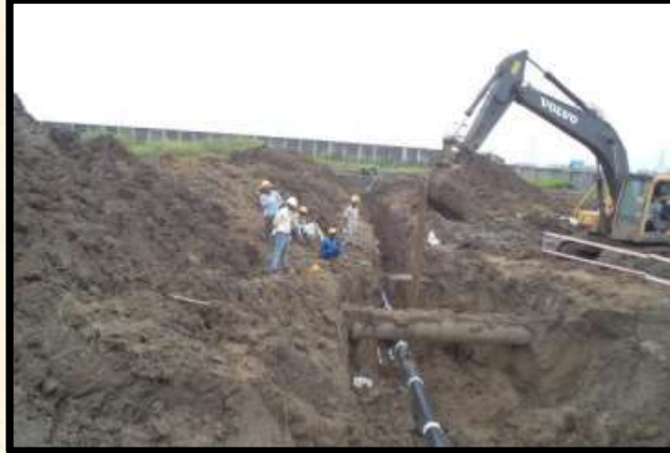
Vijaipur - Kota 16" Cross Country Pipeline Project of GAIL
