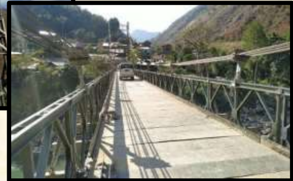
400 ft. Span Bailey Suspension Bridge over over River Kamla at Tamen for Arunachal Pradesh PWD
