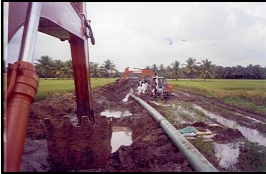
Cross Country Pipe Line Project at GAIL / KG Basin
