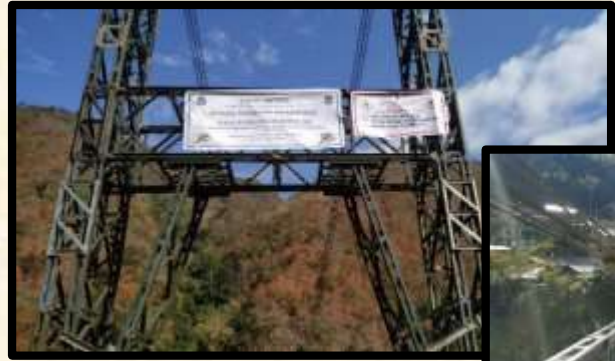
Supply, Fabrication and Erection of world's longest Bailey Bridge of 1400 ft. span, 'Col. Chewang Rinchen Setu', for Border Roads Organisation, strategically located on Shyok River between Leh and Karakoram Pass.
