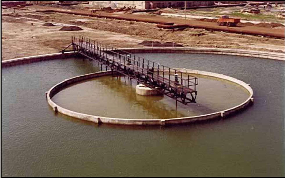
Clariflocculator with Bridge at Raw Water Treatment Plant for IPCL at Dahej
