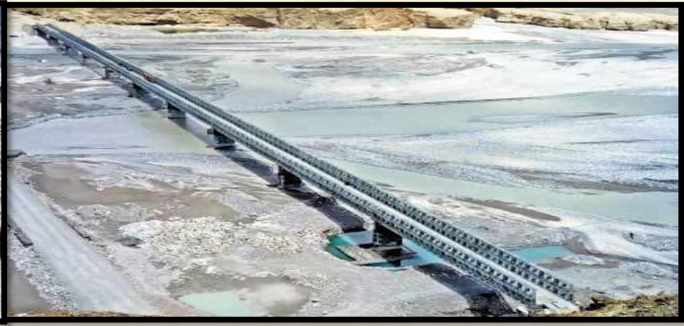
Supply, Fabrication and Erection of world's longest Bailey Bridge of 1400 ft. span, 'Col. Chewang Rinchen Setu', for Border Roads Organisation, strategically located on Shyok River between Leh and Karakoram Pass.
