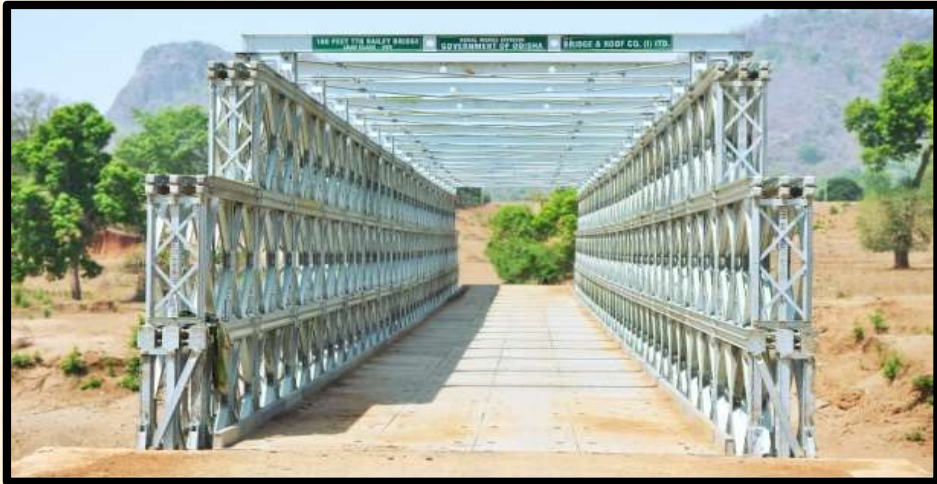
95 Nos. Bailey Type Unit Bridges including approach roads at different locations Govt. of Odisha.
