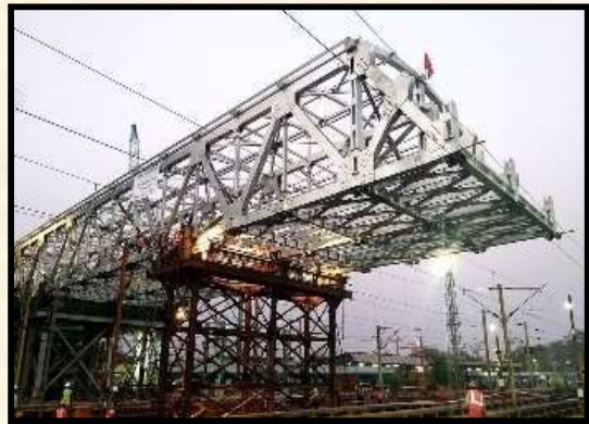
Foot Over Bridge – 3 x152 Mtr. ,12 Mtr. Wide at Santragachi Station for South Eastern Railway
