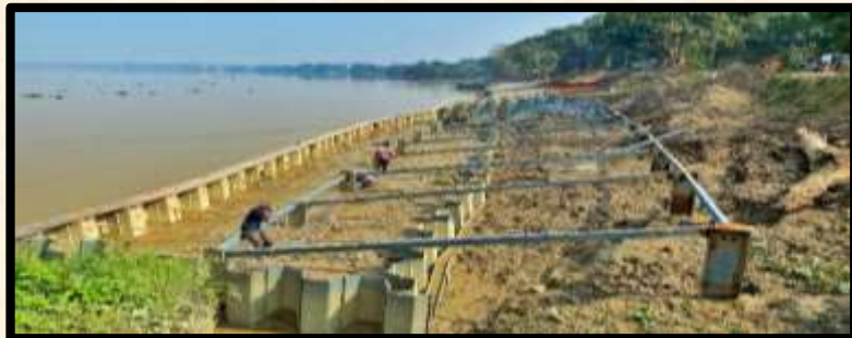
Sheet Pile & ISMB Driving
