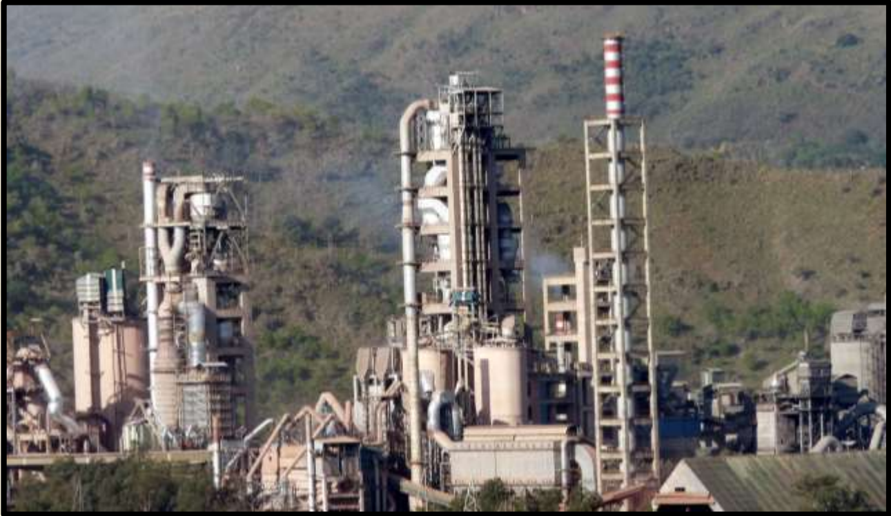
80 M High & 26 M dia. Blending Silo, 90 M high Pre-heater building at Gagal Cement Works 1 MTPA Expansion Plant for Associated Cement Co. Ltd.
