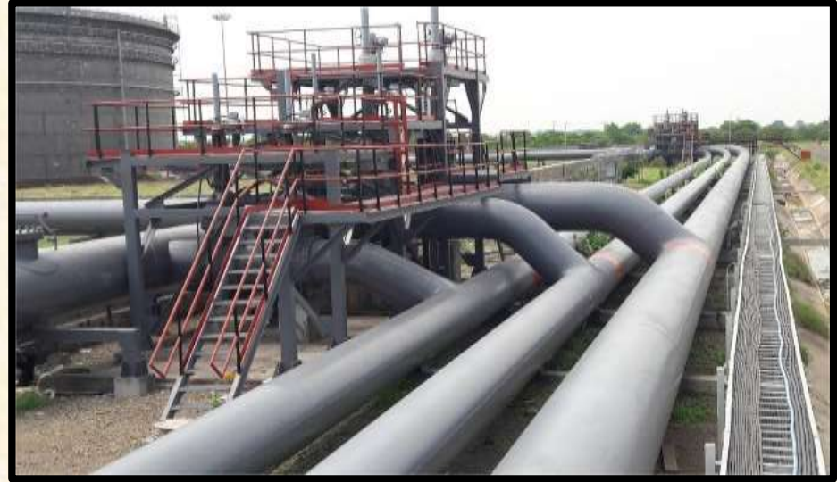
Mechanical Work at BORL Bina Terminal
