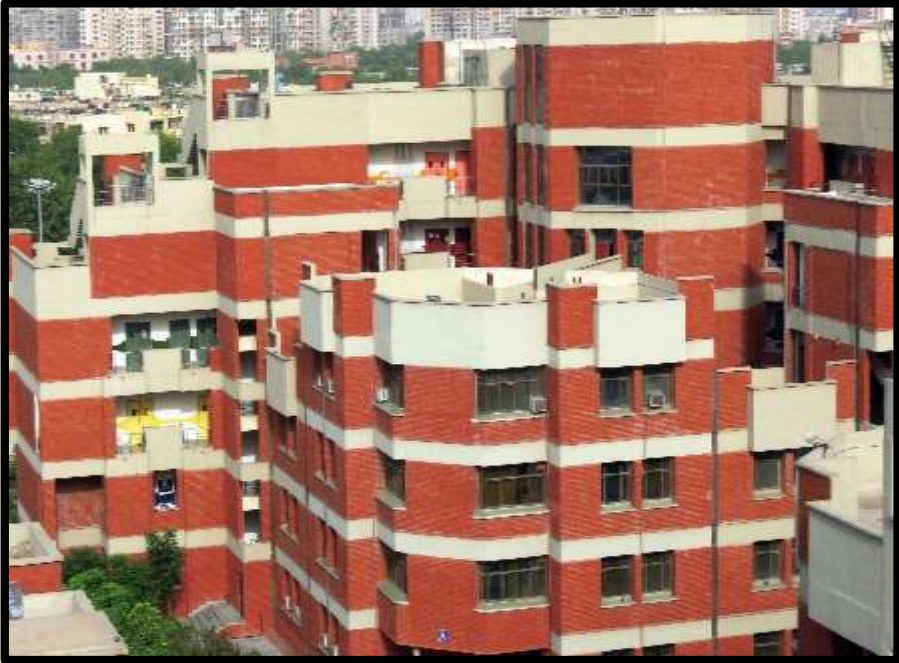
Construction of Administrative Block (G-3), Library Blocks, Academic Blocks at Guru Govind Singh Indrapastha University, Delhi
