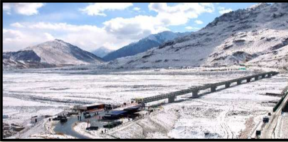
Supply, Fabrication and Erection of world's longest Bailey Bridge of 1400 ft. span, 'Col. Chewang Rinchen Setu', for Border Roads Organisation, strategically located on Shyok River between Leh and Karakoram Pass.
