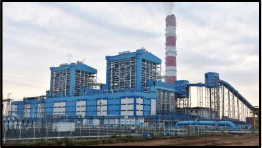
Main Power House Unit 1 including 275m height Chimney at NTPC Ltd. 2X800 MW Super Thermal Power Project at Gadarwara
